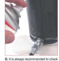
leaks on all connections to and from the cylinder by using the special gas detector
